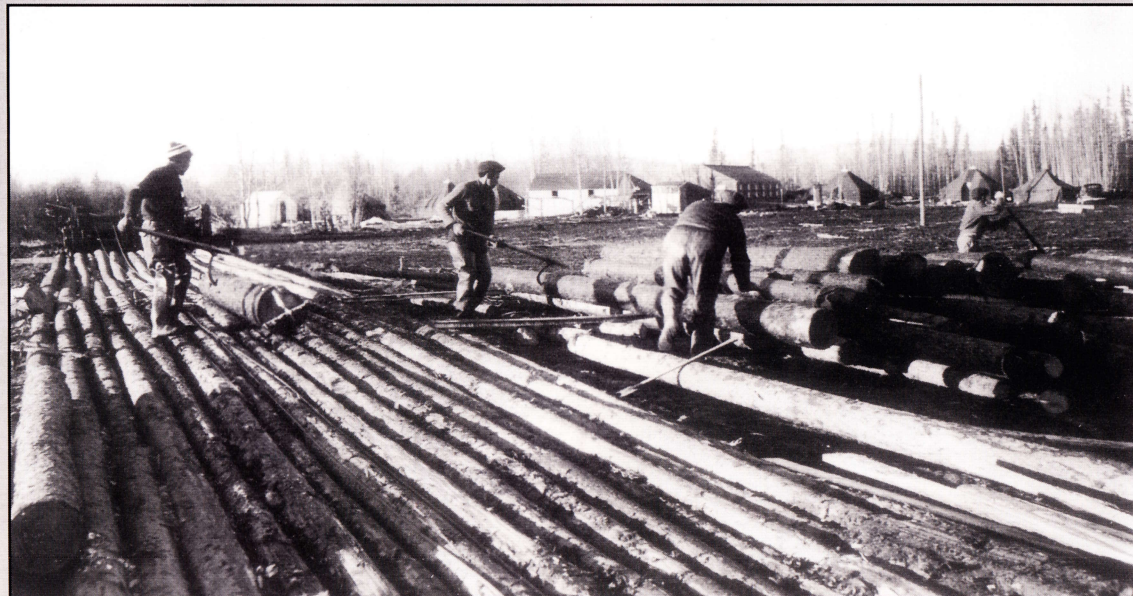
ABOVE: When the military moved into the Northway-Tanacross area, they required a prodigious amount of lumber for wartime construction. This photo shows the skidways at the Tok River sawmill. Behind the man at far left is the "donkey" that winched the logs out of the water and up the skidway; cables used to pull the logs can be seen at the man's feet. At least three of these men are Natives, probably from either Tanacross or Tetlin. Large piles of rotting slabs from the mill can still be seen in the area. (Courtesy of Lavell Wilson)
