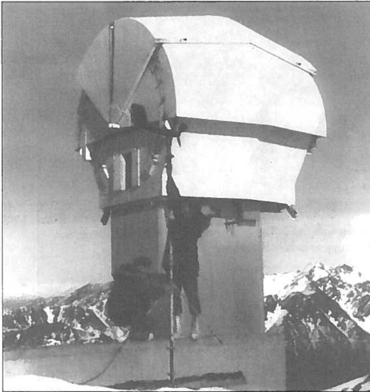
Figure 16: Soldiers perform maintenance on radar, Site Summit. Note closed clamshell covers. U.S. Army photo.
