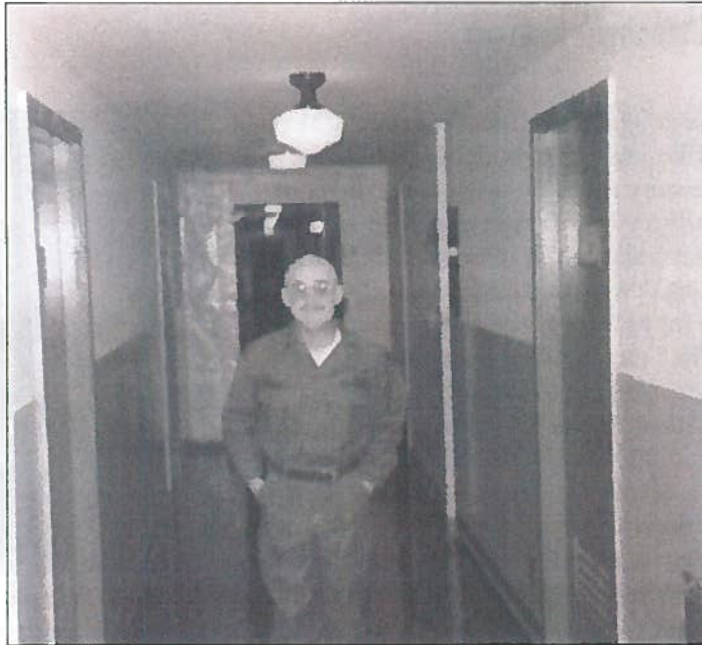
Figure 34: Soldier in hallway, Site Summit. IFC Building. Courtesy Billy Sparks.
