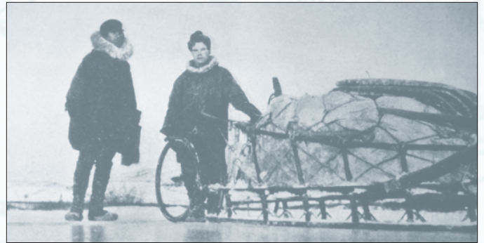
Goodwin expedition measuring the Seward to Nome route with cyclometer attached to a dogsled.
