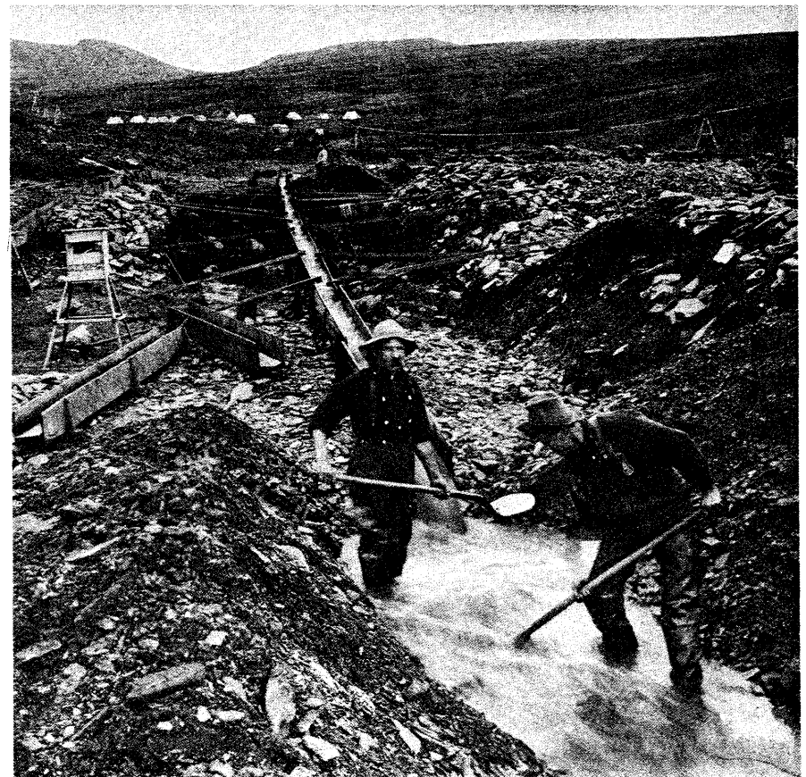
Sluicing paydirt near Nome
