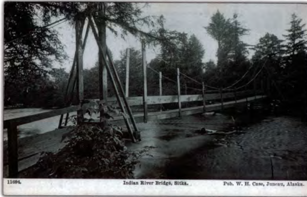
Figure 29: One of the many bridges to span the Indian River, this suspension bridge was built in 1888.
