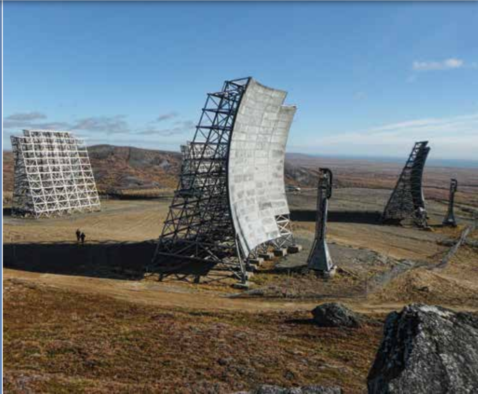
DISTANT EARLY WARNING (DEW) LINE ANTENNAS NEAR NOME, ALASKA, CA. 2013, REBECCA SHAFFER, NATIONAL PARK SERVICE, ALASKA REGIONAL OFFICE.
