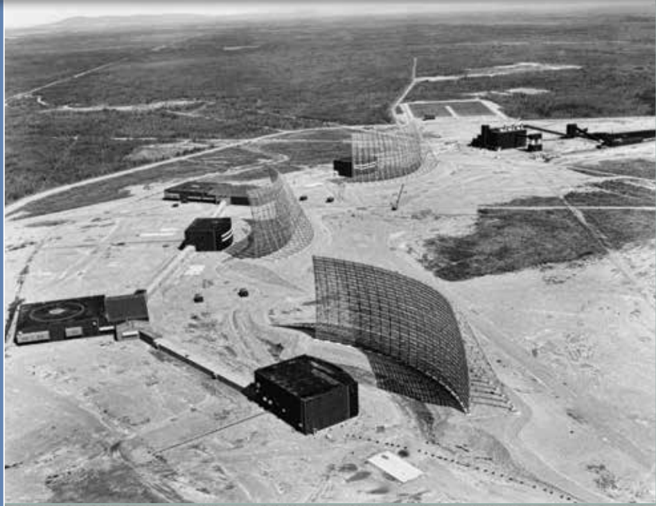
AERIAL VIEW OF CLEAR AIR FORCE STATION, BALLISTIC MISSILE EARLY WARNING SYSTEM SITE (BMEWS), CA. JULY 5, 1962, LIBRARY OF CONGRESS PRINTS AND PHOTOGRAPHS DIVISION, HABS/HAER/HALS COLLECTION.
