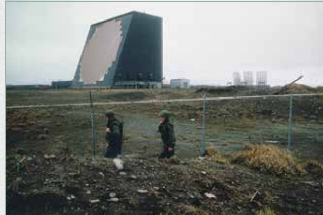
THE AN/FPS-108 COBRA DANE RADAR SYSTEM ON SHEMYA ISLAND BECAME OPERATIONAL IN 1977 AND WITH NUMEROUS UPGRADES CONTINUES TO OPERATE. DURING THE COLD WAR THE COBRA DANE RADAR SYSTEM CARRIED OUT THREE CRITICAL MISSIONS: DATA COLLECTION FOR BALLISTIC MISSILE TREATY VERIFICATION, EARLY WARNING, AND SPACE SURVEILLANCE. AMAZINGLY, WHILE COBRA DANE HAS UNDERGONE VARIOUS HARDWARE AND SOFTWARE UPGRADES, THE RADAR FRONT END, AS PICTURED HERE OCTOBER 23, 1984, HAS NOT BEEN REPLACED, USAF PHOTOGRAPH, HTTP://COMMONS.WIKIMEDIA.ORG/WIKI/FILE%3ACOBRA_DANE_SECURITY_PATROL.JPG
