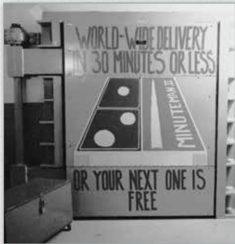
BLAST DOOR, AS PAINTED BY AIR FORCE PERSONNEL, AT THE LAUNCH CONTROL FACILITY, ELLSWORTH AIR FORCE BASE, DELTA FLIGHT, LIBRARY OF CONGRESS, HISTORIC ENGINEERING SURVEY, HAER SD-50-A-87.
