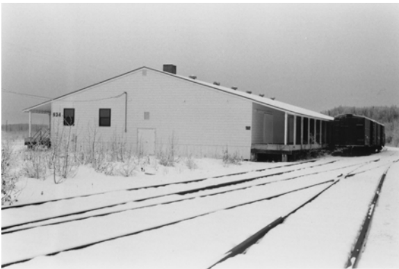
Figure 8.6 Building 934, General Purpose Warehouse, near the railroad tracks (photo by Jeff Blythe).
