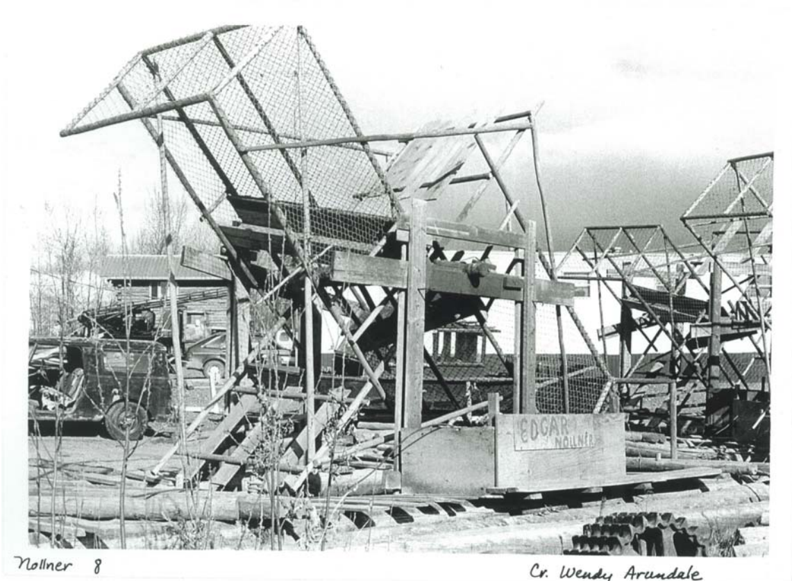
Edgar's fish wheel, hauled out on the bank in Galena, waiting for the fishing season.
