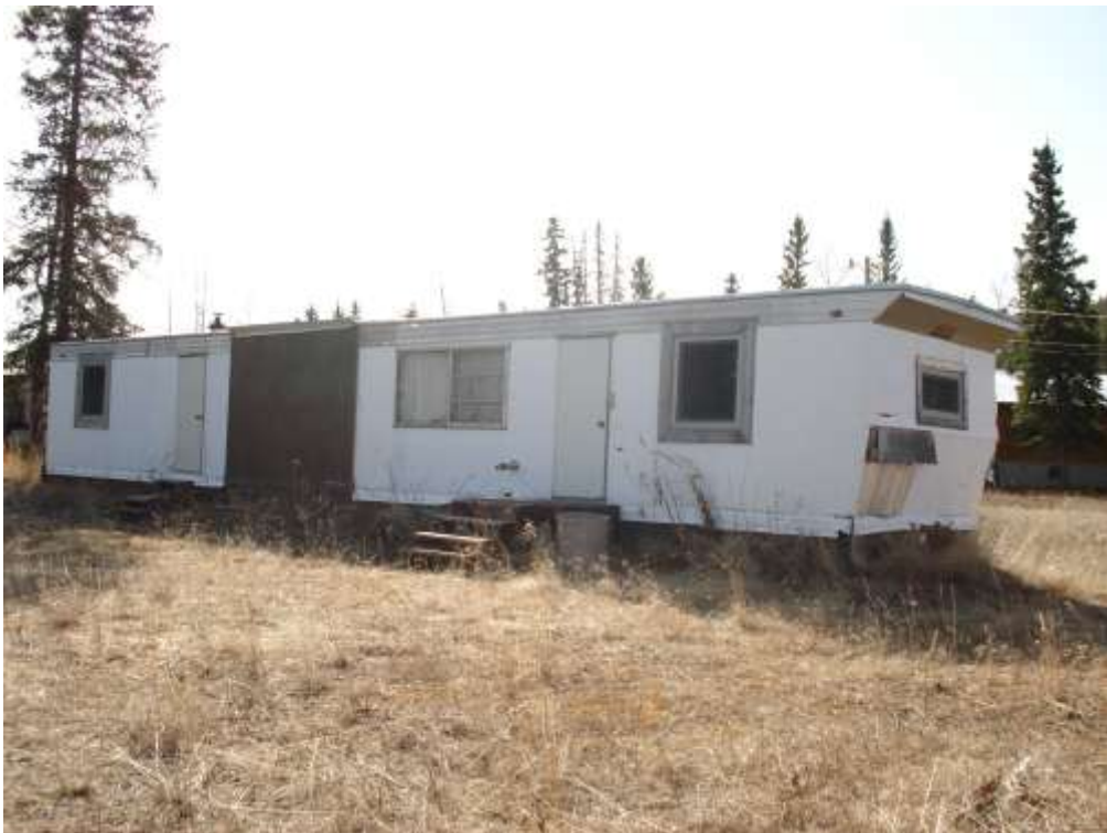
ONE OF THE VACANT MOBIL HOMES
