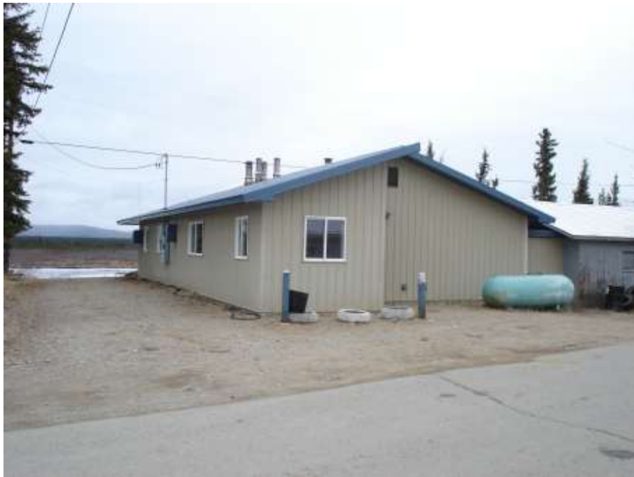
VILLAGE UTILITY BUILDING
