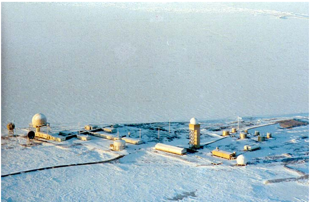
Bullen Point Short Range Radar Site (formerly Distant Early Warning Site POW-3)
