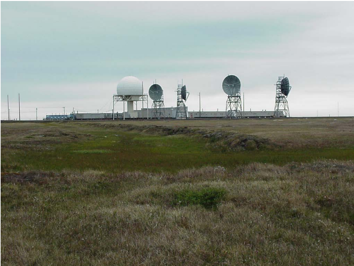
Point Barrow Long Range Radar Site (formerly Distant Early Warning Site POW-M)
