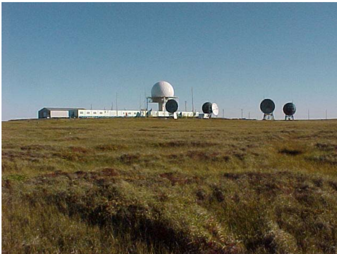
Point Lay Long Range Radar Site (formerly Distant Early Warning Site LIZ-2)
