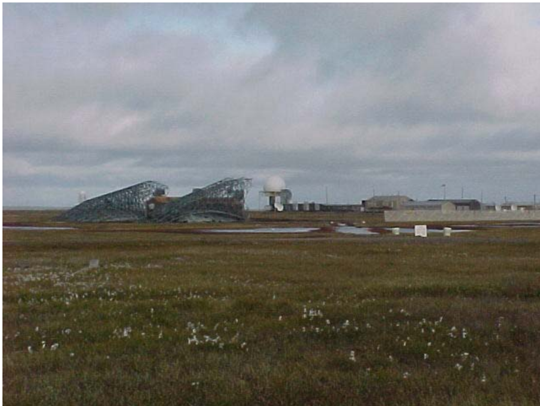
Barter Island Long Range Radar Site (formerly Distant Early Warning Site BAR-M)
