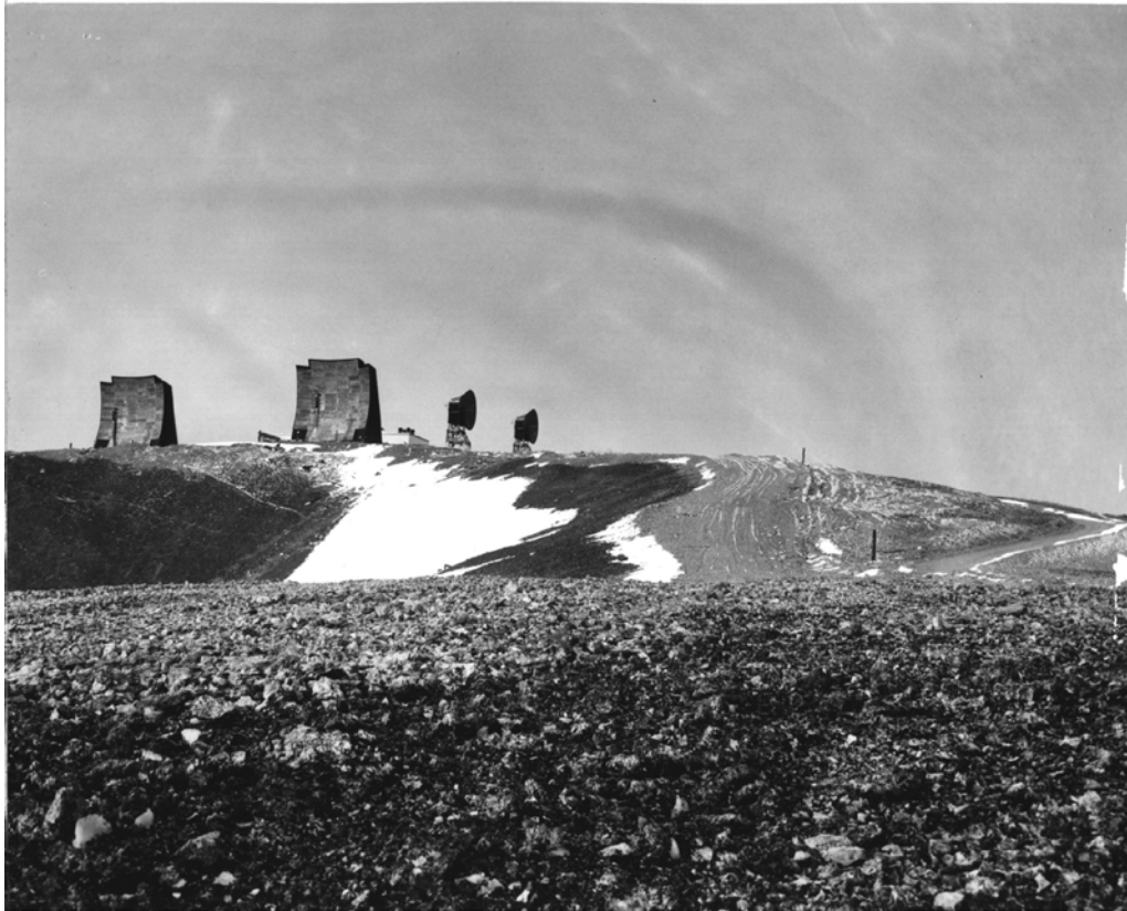
White Alice dish and tropo antennas at Cape Lisburne (Source: 11 AF archives).
