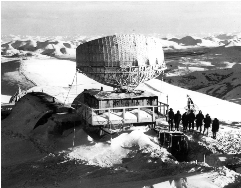
A typical early AC&W radar installation without a protective radome - probably the AN/CPS-5 at Sparrevohn circa 1951. Radar antenna were housed in radomes to protect them from powerful winds, ice, and snow (Source: 11 AF archives).
