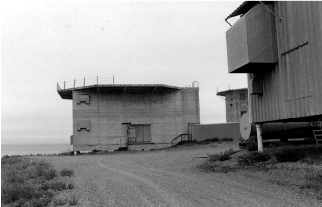
Kotzebue AC&W Site. Old radome foundation structure (circa mid-1990s) (Source Argonne National Laboratory).
