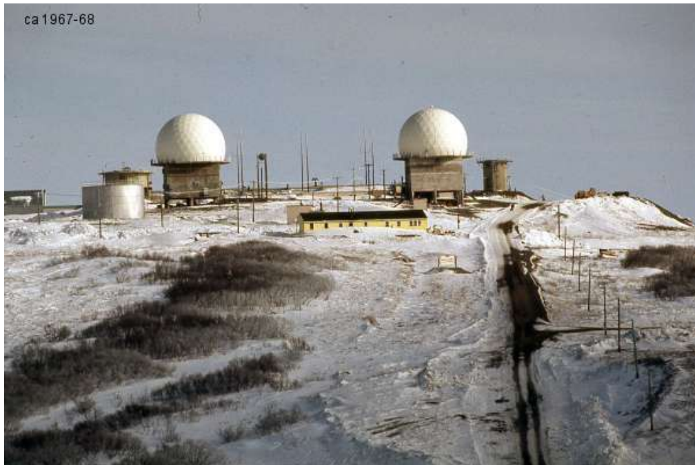
Unalakleet AC&W Site (1967-68). (Source: Online Air Defense Radar Museum).
