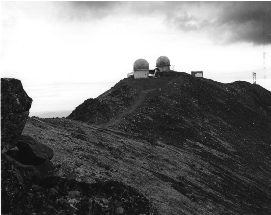
Tatalina AC&W Site (undated). Photograph showing the top camp and the two radomes, the parabolic antenna from the White Alice Communication System (to the right), and the cable tower from the tramway (Source: 11 AF archives).
