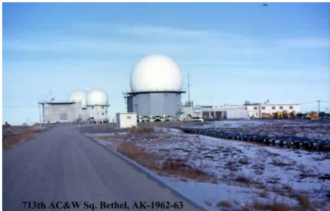
Bethel AC&W Site (1962-63). (Source: Online Air Defense Radar Museum).
