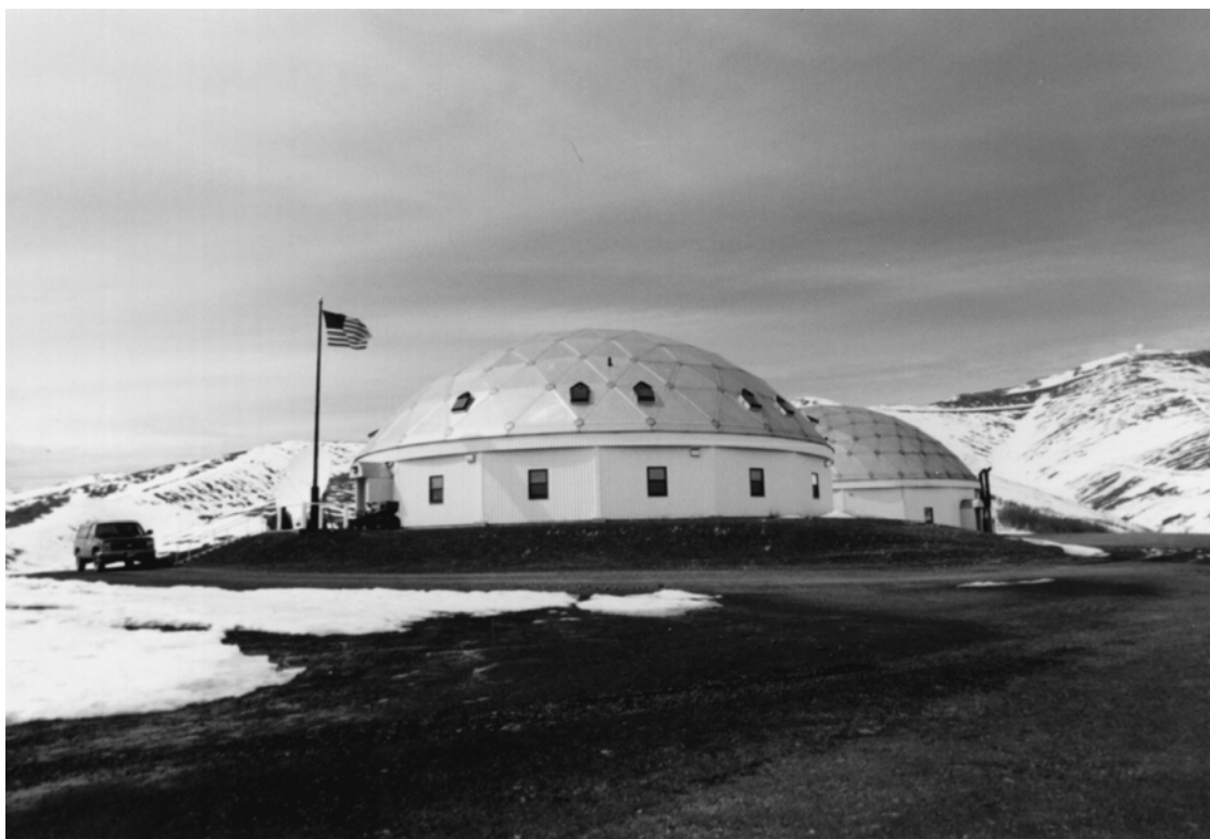
Sparrevohn Long Range Radar Site (circa 1980s) showing new, double domed composite buildings (Source: 11 AF archives).
