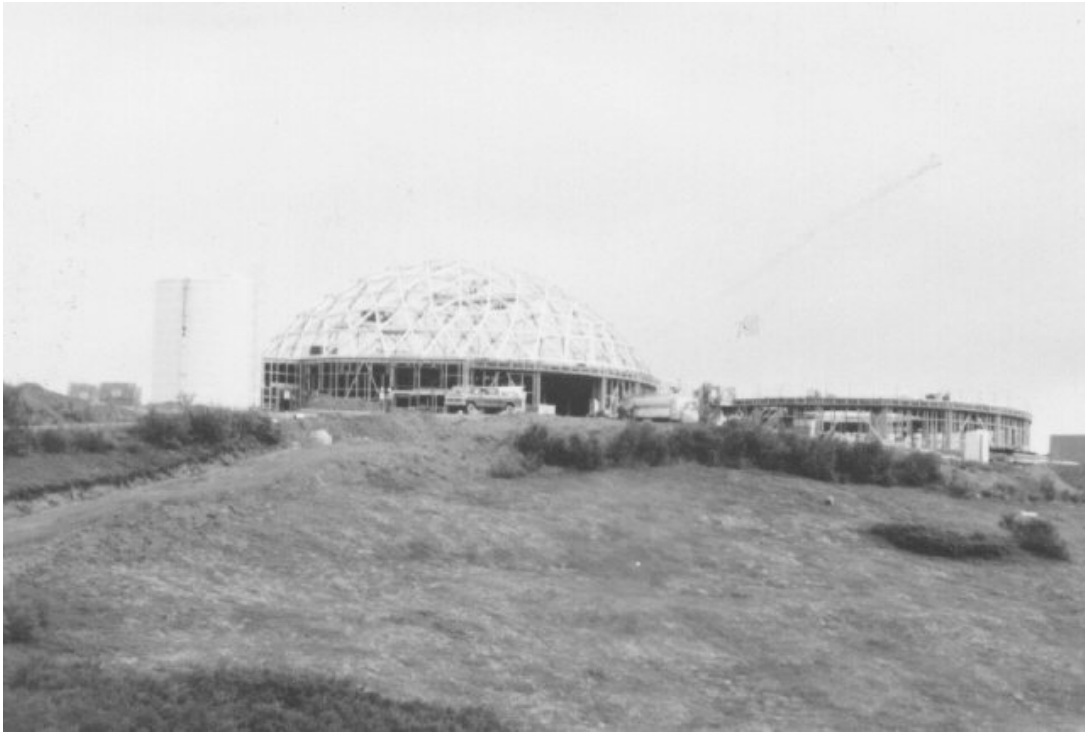
Sparrevohn LRRS (circa 1984-1984). Geodesic Dome Construction (Source 11 AF archives).
