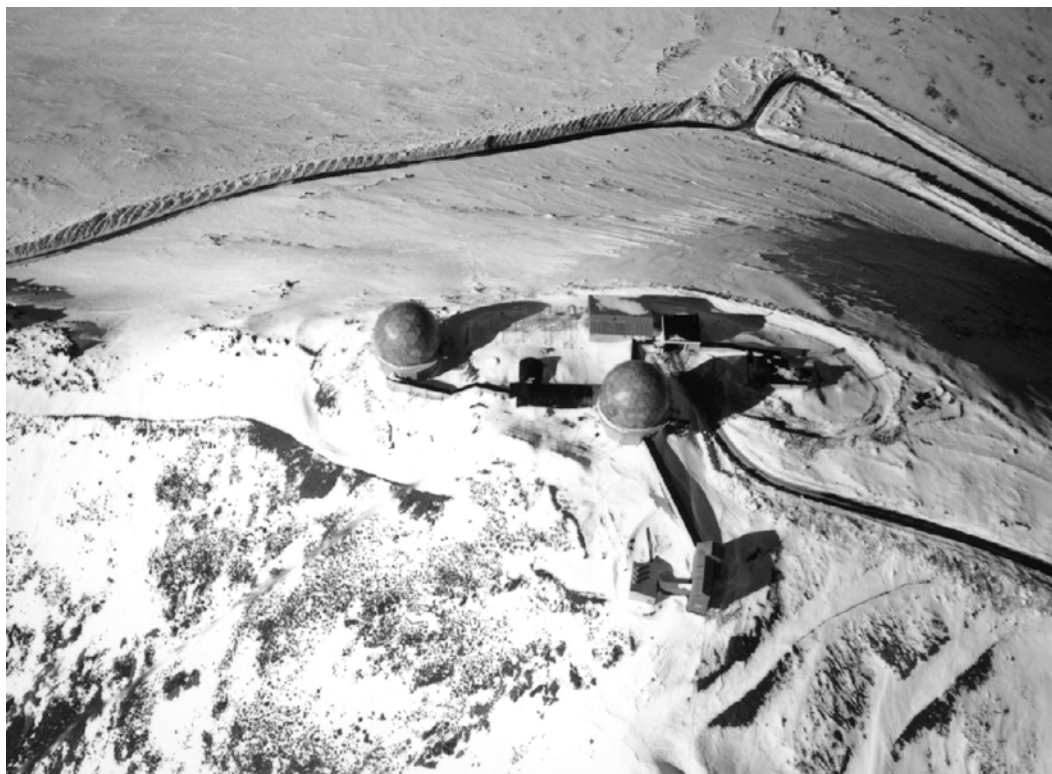
Tatalina (circa 1950s). Aerial view showing a typical AC&W station layout. The radomes, support buildings, and connecting passageways can be seen (Source: 11 AF archives).
