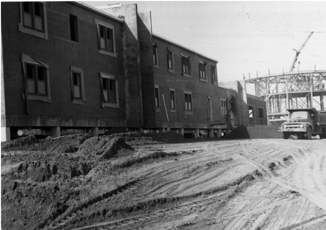
Fort Yukon AC&W Site (circa 1956). Construction of Officers Quarters showing how early buildings were wood and one or two stories high (Source: 11 AF archives).
