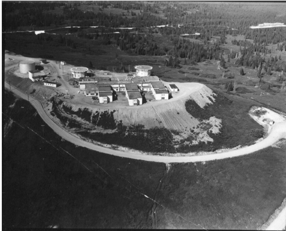
Ohlson Mountain AC&W Site (undated) showing the radome foundation structures without the protective domes or antennas in place (Source: 11 AF archives).
