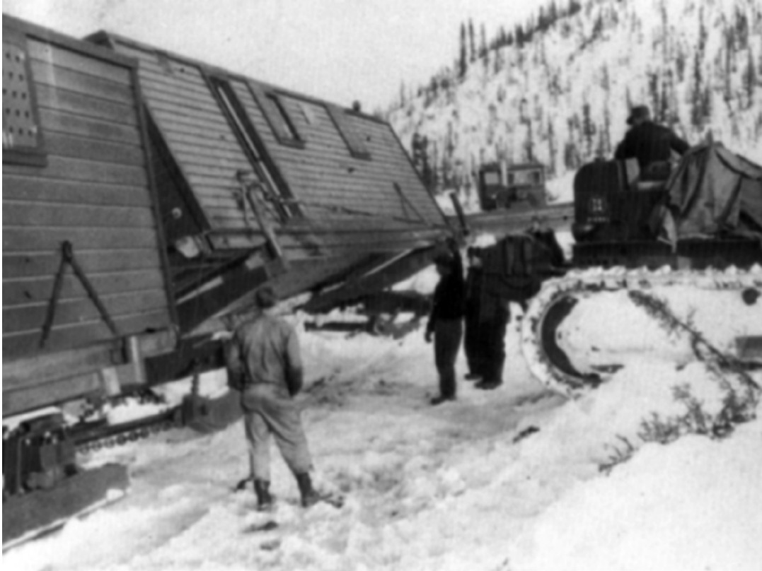
Modular building construction, circa 1950s, at an unknown site. Modular buildings allowed more rapid field construction during the shortened field season (Source: 11 AF archives).
